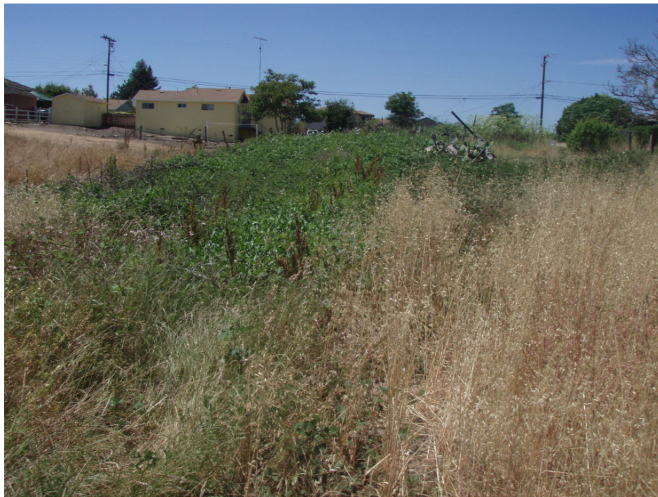
Photo 2. Upstream section of drainage swale.
